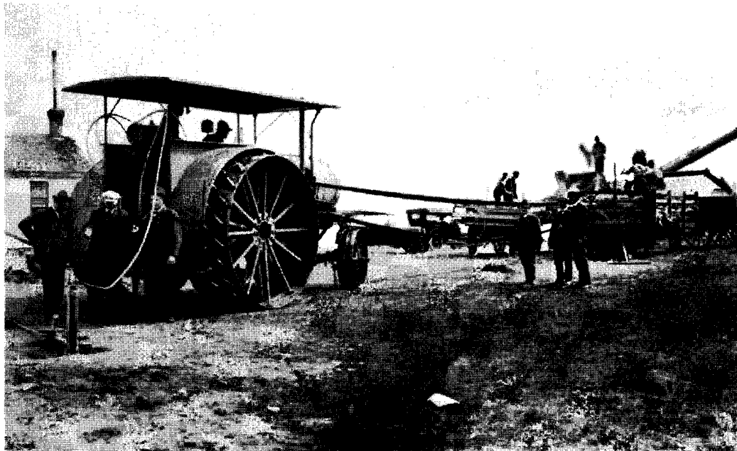
Figure 6. Threshing scene in 1919 near Mohall, North Dakota. A 60 hp gasolene engine is pulling a 42" separator, the engine being operated by natural gas from the wellhead at left.
