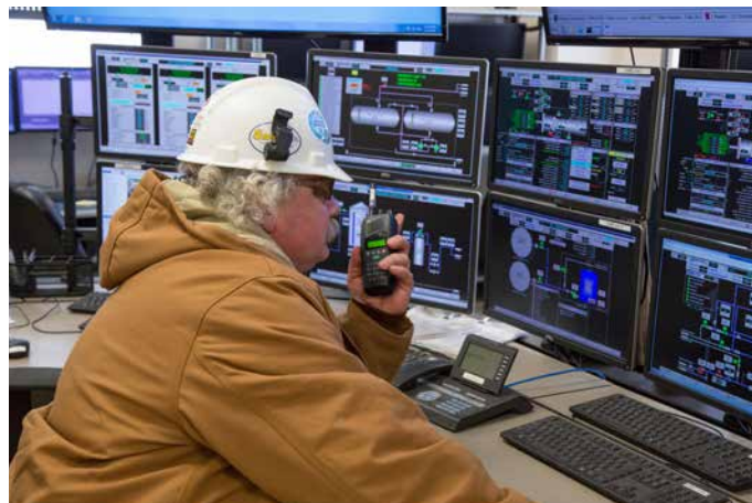
+ Donald Drake, an operator-technician, is shown in the control room at the Lonesome Creek Station, near Watford City, N.D. The station consists of five, 45-megawatt capacity generating units. The plant is owned by Basin Electric Power Cooperative, Bismarck, N.D. Photo courtesy of Basin Electric.
