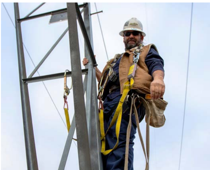
+ Wayne Bentz, lead lineman from Basin Electric Power Cooperative's Menoken Transmission System Maintenance outpost, is a graduate of Bismarck State College's Lineman program. Photo courtesy of Basin Electric.
