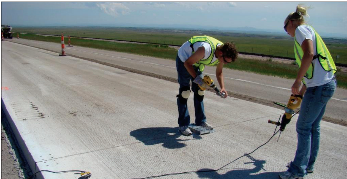
SDSU graduate students installing joint instrumentation on U.S. Highway 212 west of Belle Fourche, SD.
