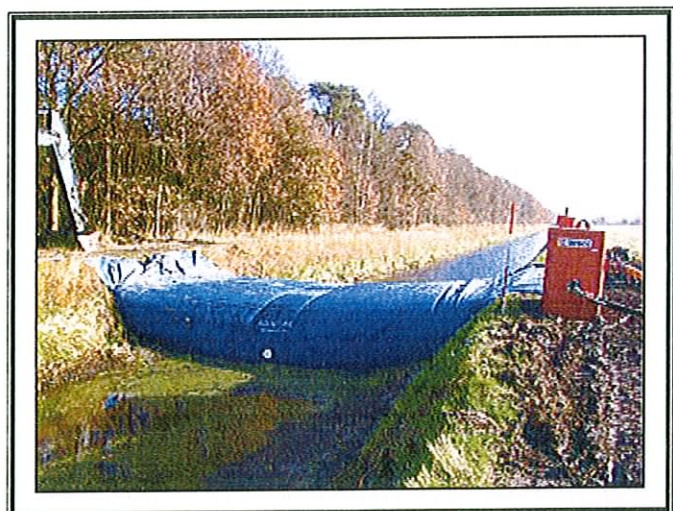
Figure 2.3 Inflatable Cofferdam
