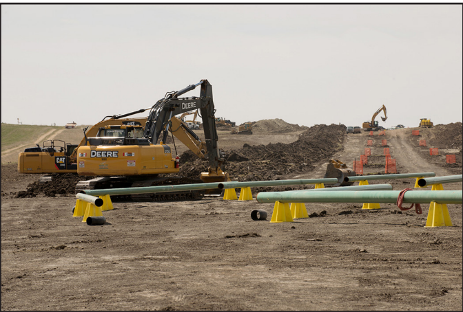
Construction of Watford City bypass, May 2014
