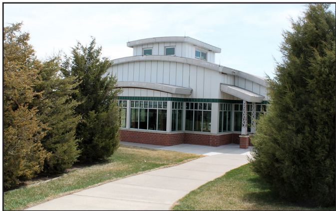
East bound I-94 Hailstone Creek Rest Area near New Salem.
