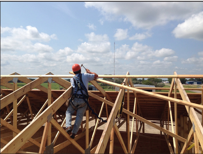
Construction of new salt shed in Minot District.
